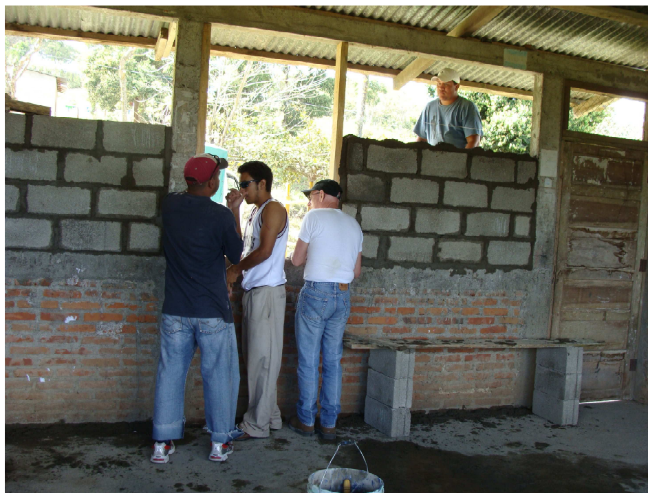
Remodeling a school in Saraguasca
